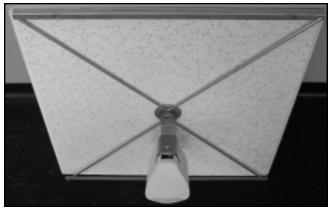
Step 4: Attach a 40-4082 or 40-4083 speaker to metal speaker plate and support bar. Secure to speaker with supplied screw.
