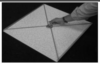
Step1: Place the metal bracket over the ceiling tile and push the support pin through the bracket and tile.
