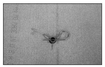
Step 3: Secure support pin to ceiling tile with lock key.
